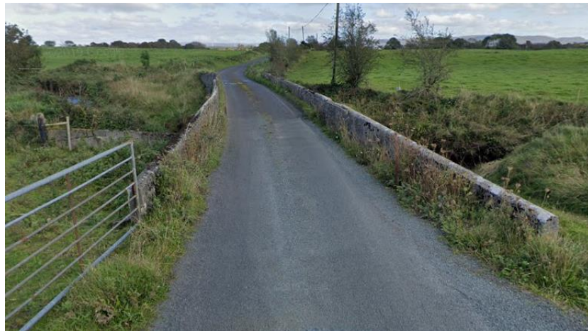
Photo 15.5 – Bridge along Local Road L-6612
