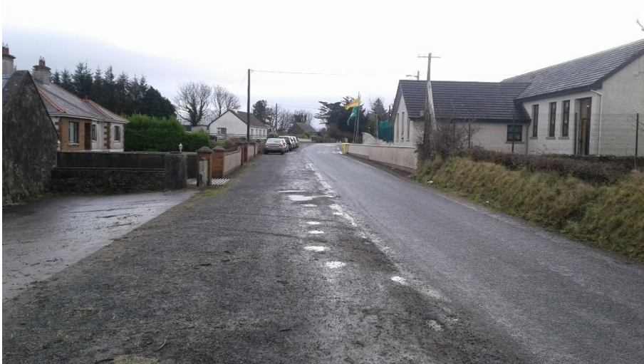
Photo 15.2 – Local Road L-2604-0 – Stokane National School
