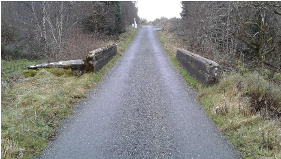
Photo 15.3 – Local Road L-2604-0 – Bridge
